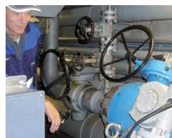
Plant Manager Markus Schuster is happy with the renewal of the isolating sections without welding works. The compact TBV design allows exchanging the old, flanged valve.
