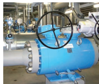
For highest safety requirements: Twin Ball Valve isolating section in extra compact design.
